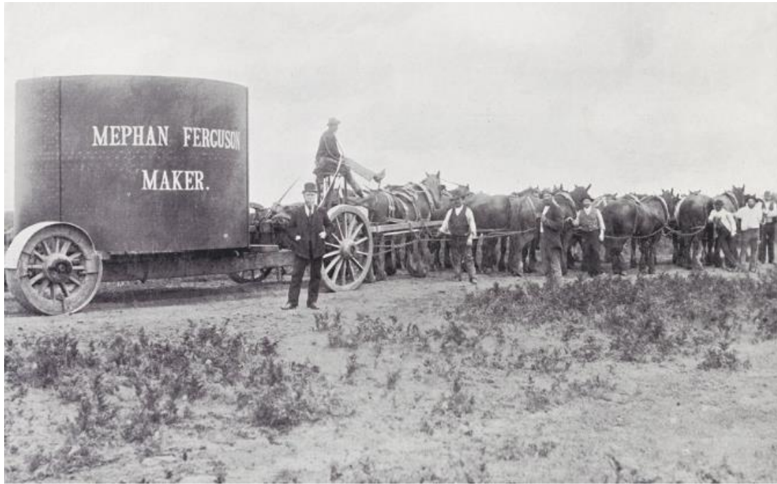
Delivery of Clark's tunnelling shield for sewer construction in bad ground, Port Melbourne, circa 1894.
